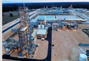
Chemours – Fayetteville, NC Air emission controls include carbon absorbers, waste gas scrubbers and a thermal oxidizer
